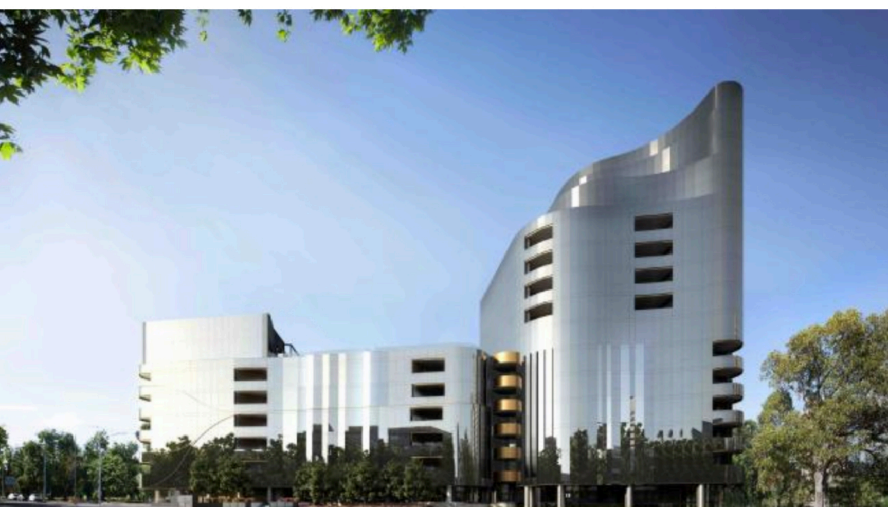
Devitt Property Group's The Muse apartment development on St Kilda Rd, Melbourne, will be fitted with top tech. Source:Supplied
